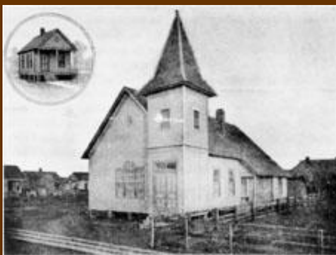
No. 13. Movable Chapel and Recent Addition.
