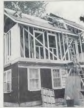
South Haven Church members came to the aid of the Schmeling family by closing off a new addition and roof before the rain came.
